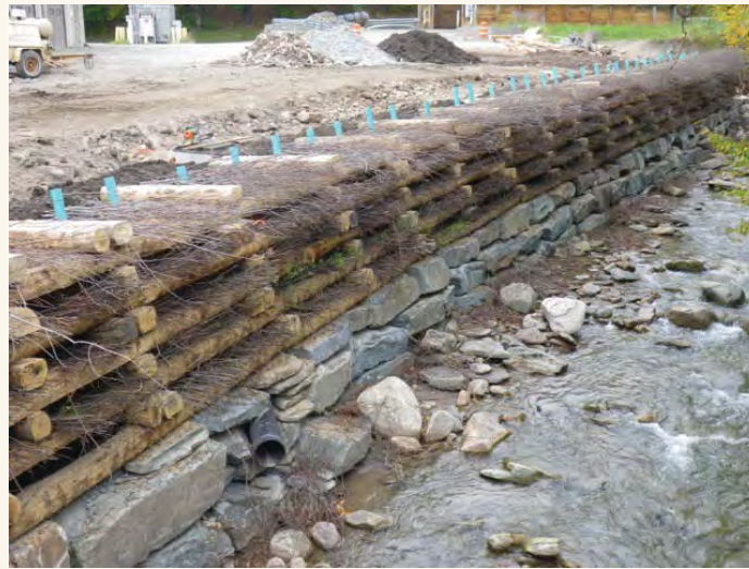
Live brush matting placed within wood cribbing
