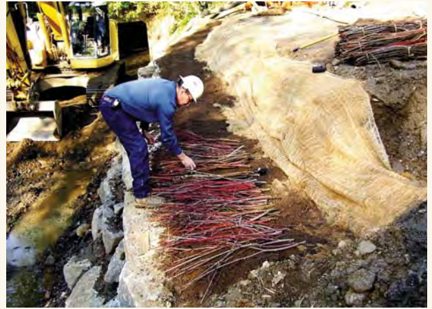
Laying of brush matting above boulder seawall
