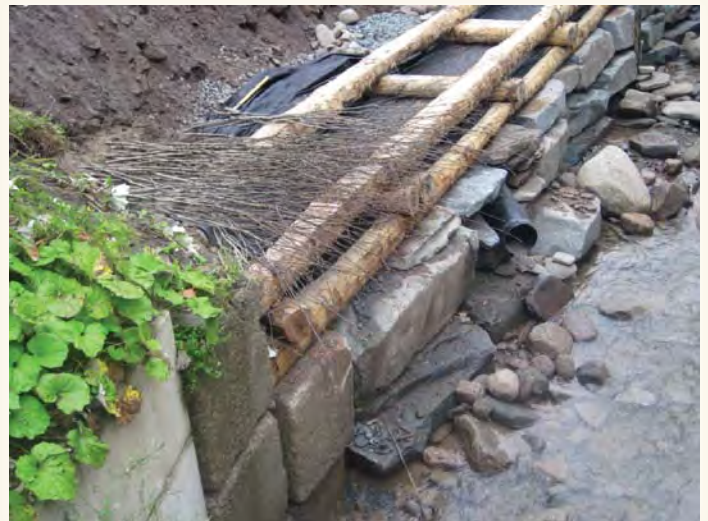
Live brush matting being placed on wood cribbing
