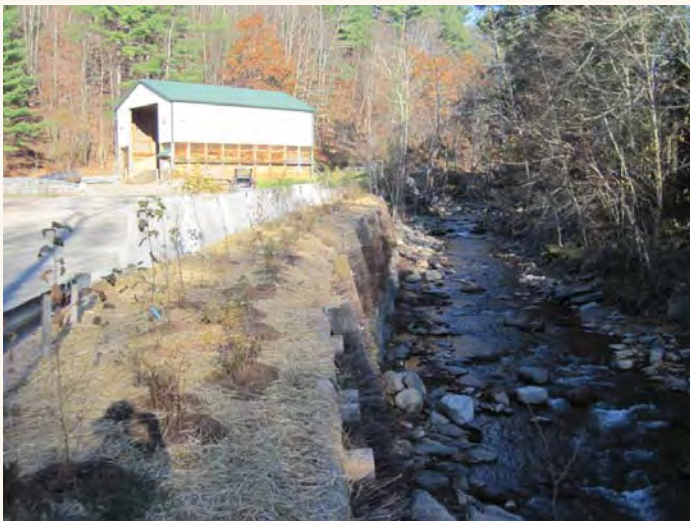
Vegetated buffer zone installed on top of wood cribbing wall
