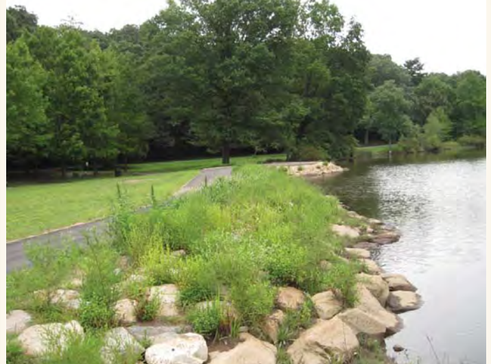
Natural boulder / native plug revetment
