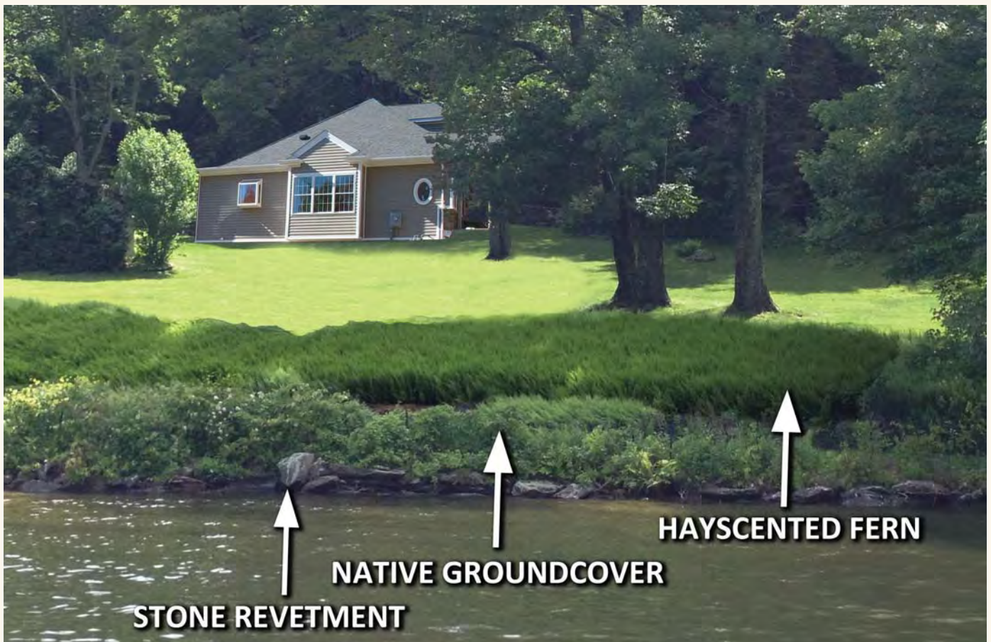
Example of naturally vegetated, stabilized shoreline using hay scented fern and native groundcovers
