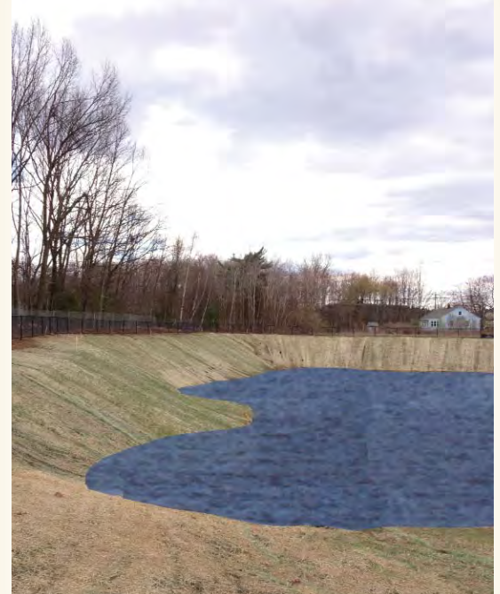
Erosion control netting placed on steep slopes stabilizes soil after grading
