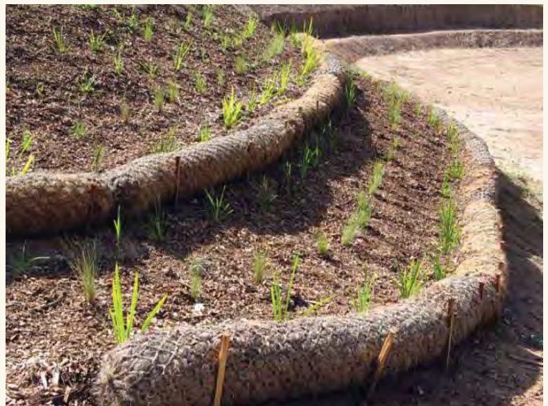
Coir logs stabilization with native plugs
