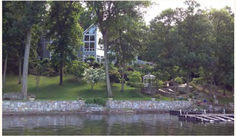
Example of stone masonry seawall
