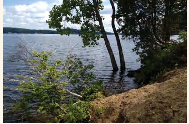
Wave action has destabilized the vegetated bank leading to erosion.
