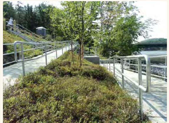
Lowbush blueberry sod used on bank to control erosion - 1 week after installation
