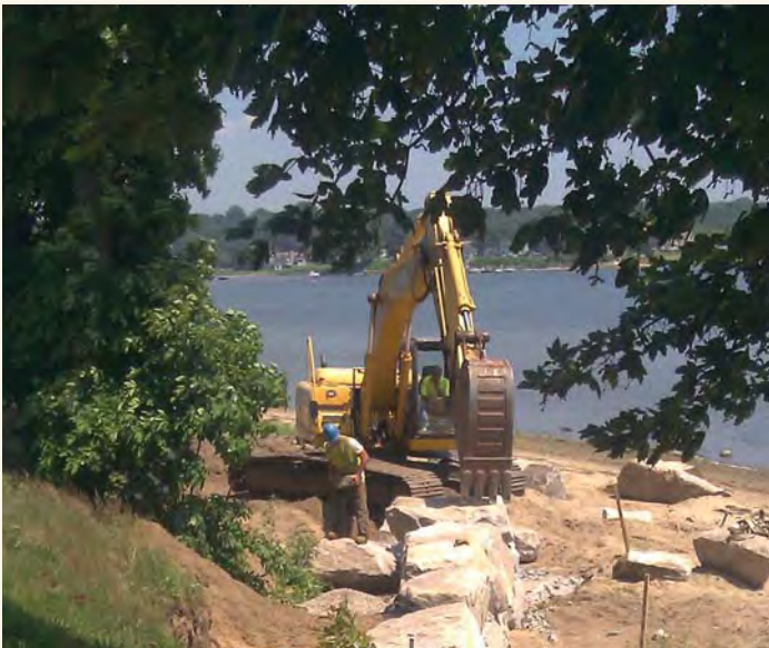
Contractor installing boulder wall revetment
