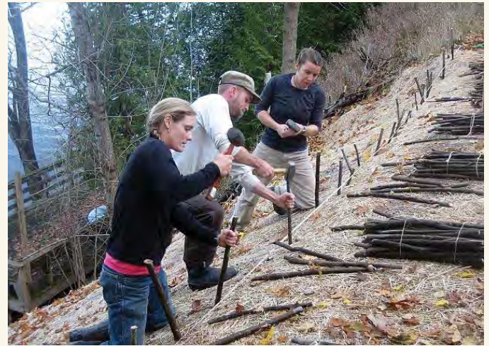
Installation of live stakes
