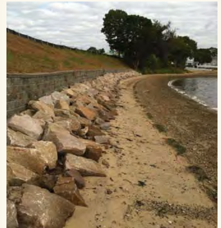
Example of Emergency Boulder Armoring Repair to Dry Stacked Block Seawall
