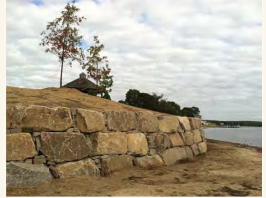
Example of dry staked boulder seawall
