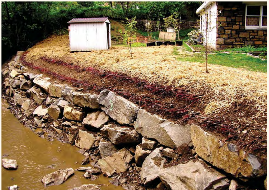
Bioengineered shoreline protection of dry staked boulders, and live fascines
